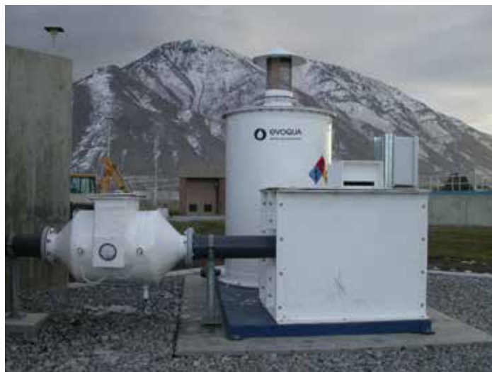
Carbon adsorption is the simplest of the vapor-phase technologies, with no required chemical storage and feed system, and no biological process to maintain. (RJC Modular Carbon Adsorber)
