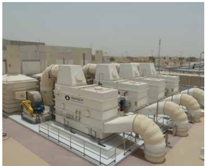
An example of a typical wet scrubber system, documented as the most reliable and flexible vapor-phase technology. (LOPRO® Odor Control System)
