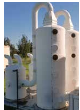
Carbon Adsorbers used as polishing units following a Biotrickling filter.
