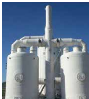
Carbon Adsorbers used as polishing units following a Biotrickling filter.
