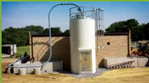
The BioMag system, pictured above, uses the inert material magnetite to add weight to biomass.
