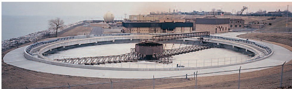
Storm water half bridge clarifier installation with walk through truss bridge.
