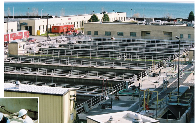
Rectangular clarification units are well suited to facilities that have a limited footprint.
