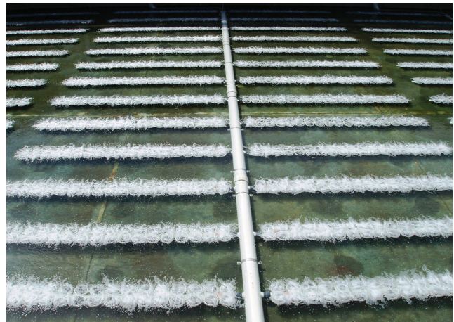
Installation of a DualAir® Membrane Diffuser System
